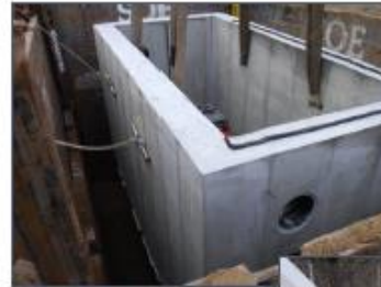
Vault Installation
